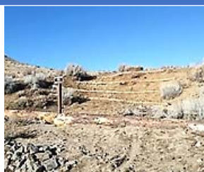
Erosion and Sediment Control
